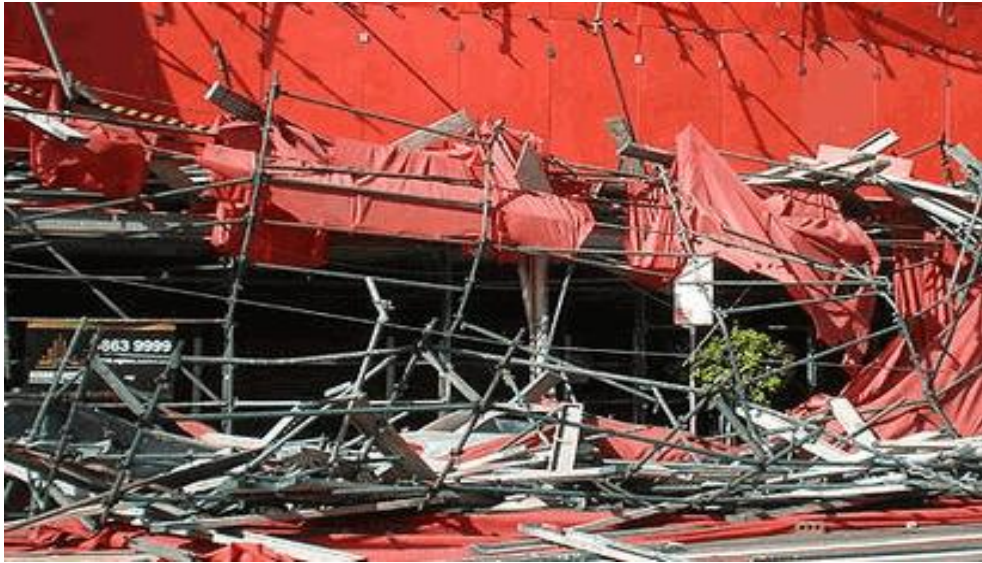
MELBOURNE - Prahran scaffolding collapse - February 24th, 2009
