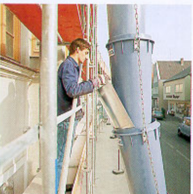
Galvanised steel chute liners protect the areas subject to severe wear and stress prolonging the chute life even further.
