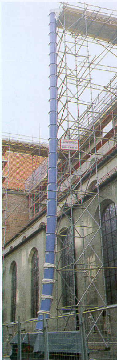
A fully tested galvanised steel chute fixing frame ensures the chute is safely secured to the scaffolding.
