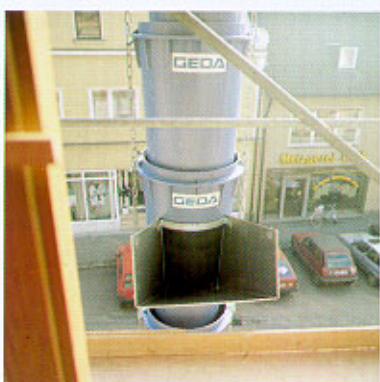
Chute branch sections are ideal for multi-level applications.
