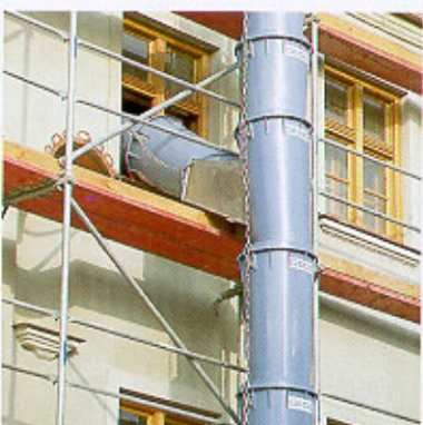
Chute branch sections are ideal for multi-level applications.
