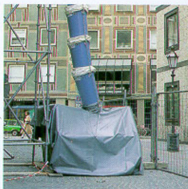
Dust protection collars eliminate dust nuisance from the chute and skip covers help retain waste material in the container.
