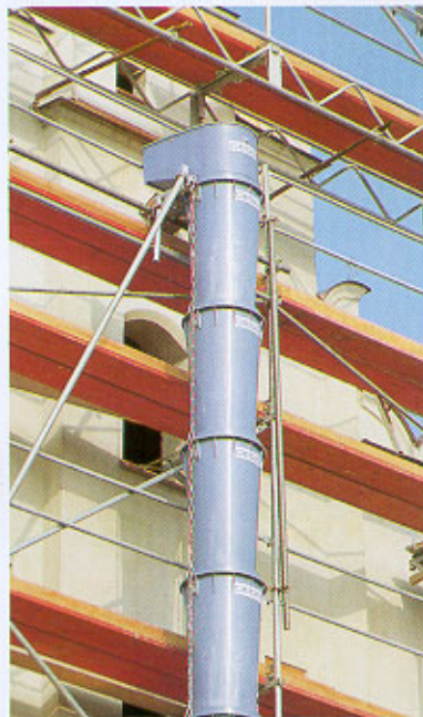
A fully tested galvanised steel chute fixing frame ensures the chute is safely secured to the scaffolding.
