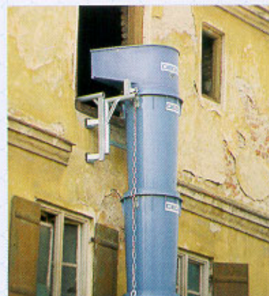
The generous dump hopper width allows easy emptying of wheelbarrows.
