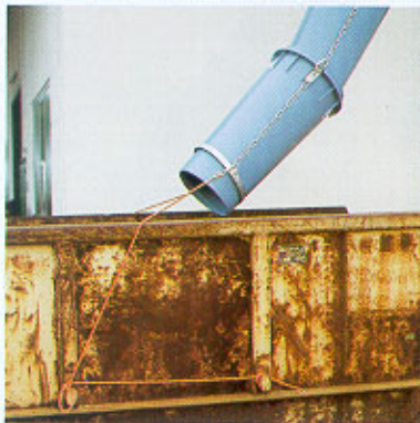
Guide ring allows the chute to be directed into a container and fixed in position with ropes attached.
