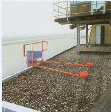
A special frame using ballast weights and incorporating verge protection allows use of chutes on flat roofs.
