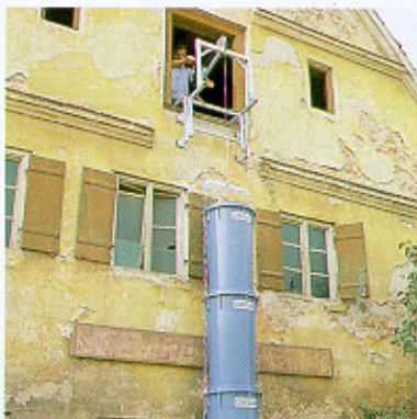
A special purpose designed hand winch is available for rapid erection and dismantling of the chute.
