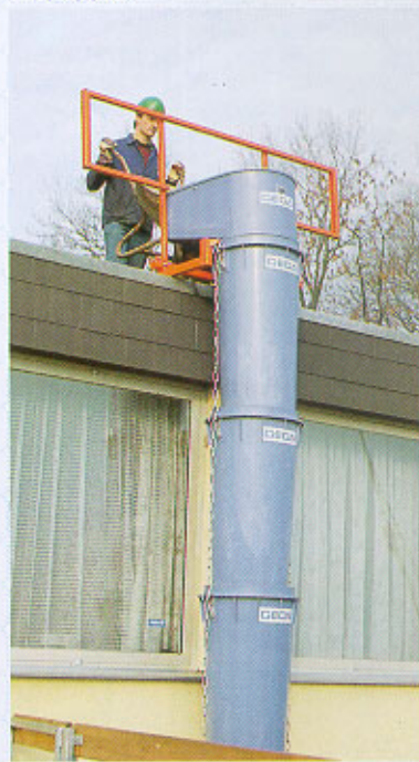
The generous dump hopper width allows easy emptying of wheelbarrows.
